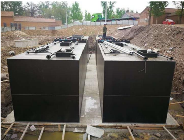
Rural sewage treatment project in Wuqing District, Tianjin
