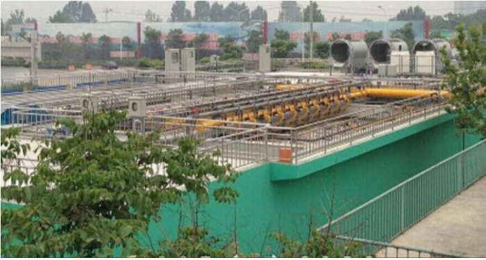
Ma'anshan Sinosteel Tianyuan Chemical Wastewater Reuse Project
